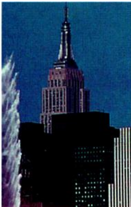
WCBS-TV's wideband antenna atop the Empire State Building may serve as an interim solution for broadcasters looking for a DTV transmission site.
